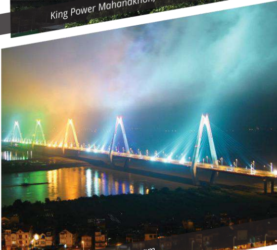
Nhat Tan Bridge, Vietnam
